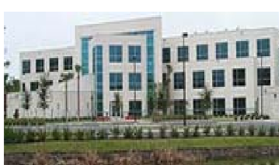
The National Center for Forensic Science Building
